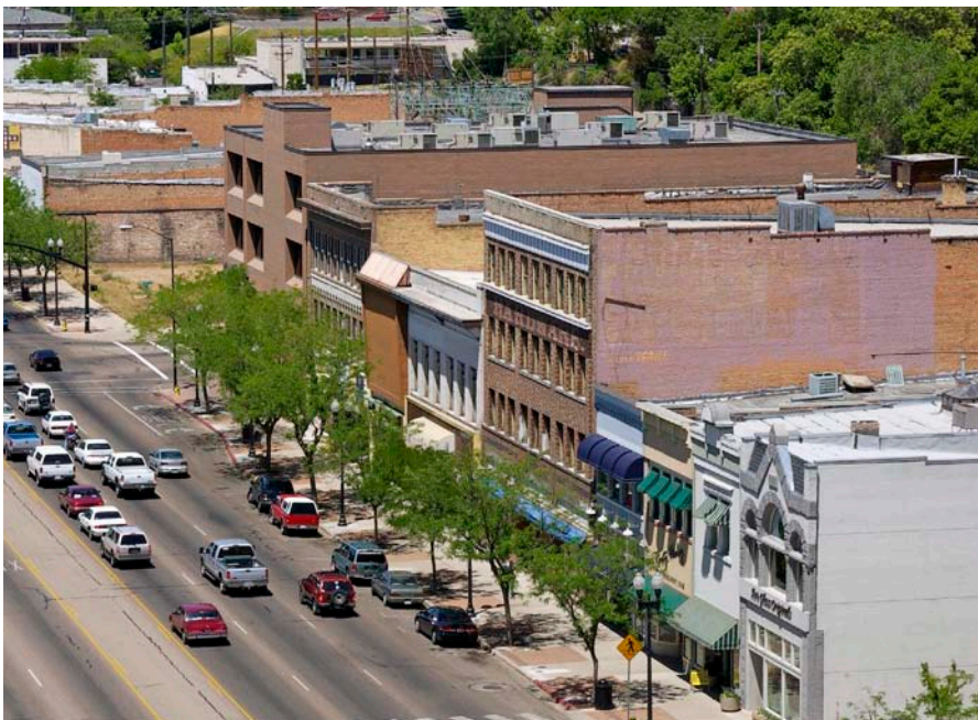
Infill development in Ogden, Utah used the framework of historic buildings to reinvigorate the downtown.
