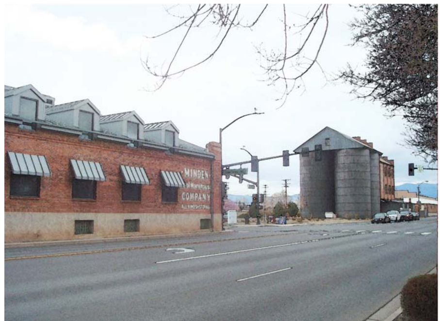
Existing view of US 395 by the Minden Flour Mill.
